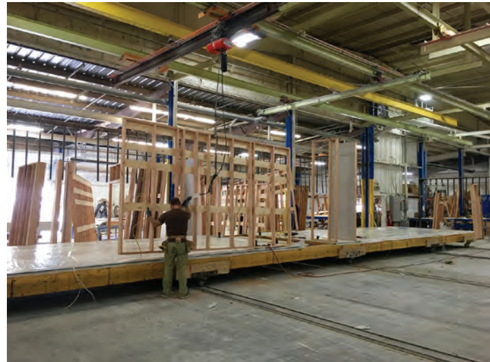
Assembly of module components in a controlled environment
