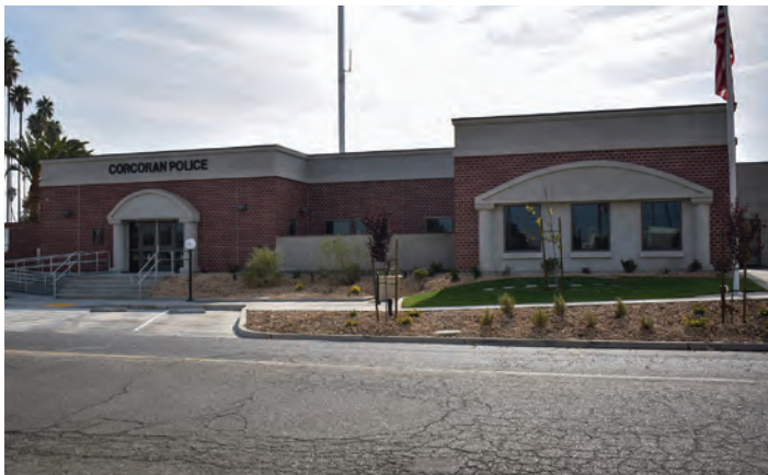
Corcoran Police Station. Built by Silver Creek Industries & Accelerated Modular Concepts, Inc. First Place: Permanent Modular Correctional.
