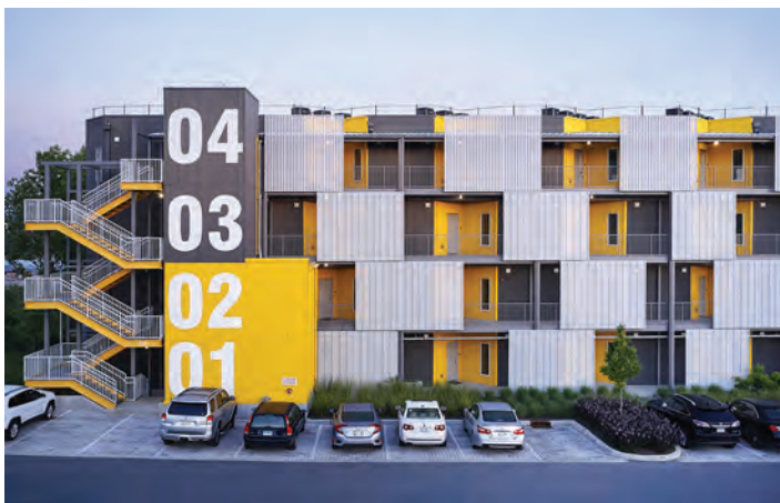
Alloy at Tech Hill (close-up). Built by Champion Commercial Structures. First Place: Permanent Modular Multifamily
