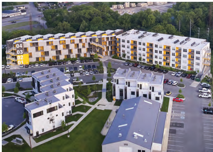
Alloy at Tech Hill (wide). Built by Champion Commercial Structures. First Place: Permanent Modular Multifamily
