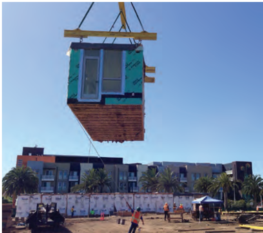
Transportation of modules to a final destination
